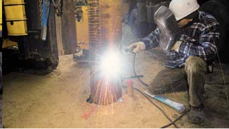
lengthening of the pipe
